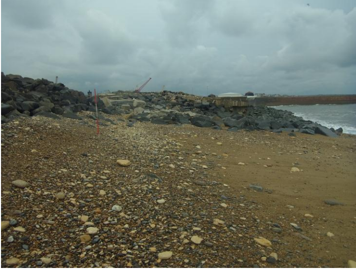
Plate 5 – Survey photograph 1bSNC4_20130911_N3.JPG (FM 2013)
