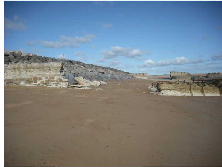
Plate 9 – Survey photograph 1bSNC6_20120918_N2.JPG (FM 2012)
