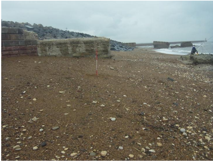
Plate 8 – Survey photograph 1bSNC6_20130911_N4.JPG (FM 2013)
