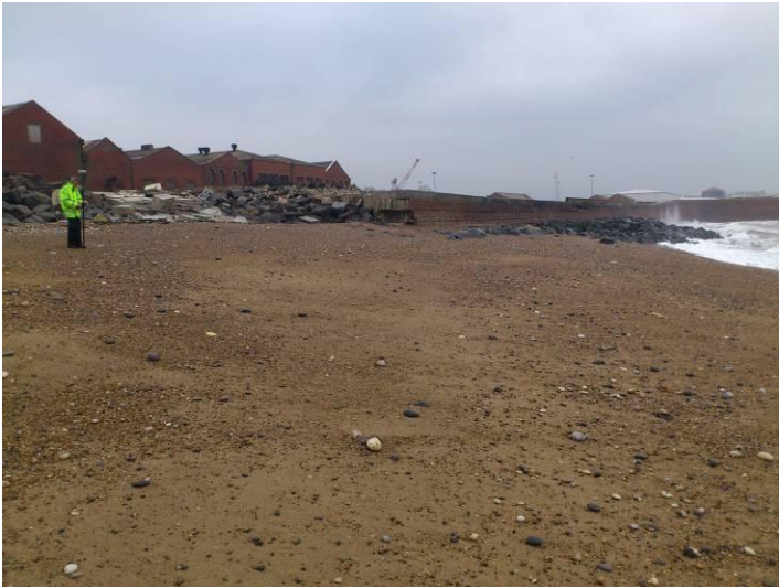
Plate 7 – Survey photograph 1bSNC4_20111111_N2.JPG (FM 2011)
